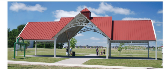
Riverside Park Pavilion
