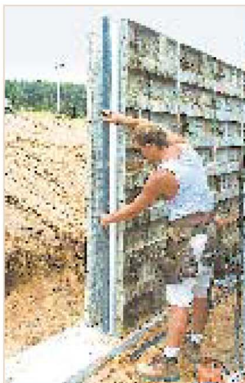
Clockwise from top: A diagram shows how the E-MAXX insulation form is constructed; a construction worker installs the form; a side view of an E-MAXX panel; the final results of the system which provides continuous insulation on one or both sides of a poured foundation.
