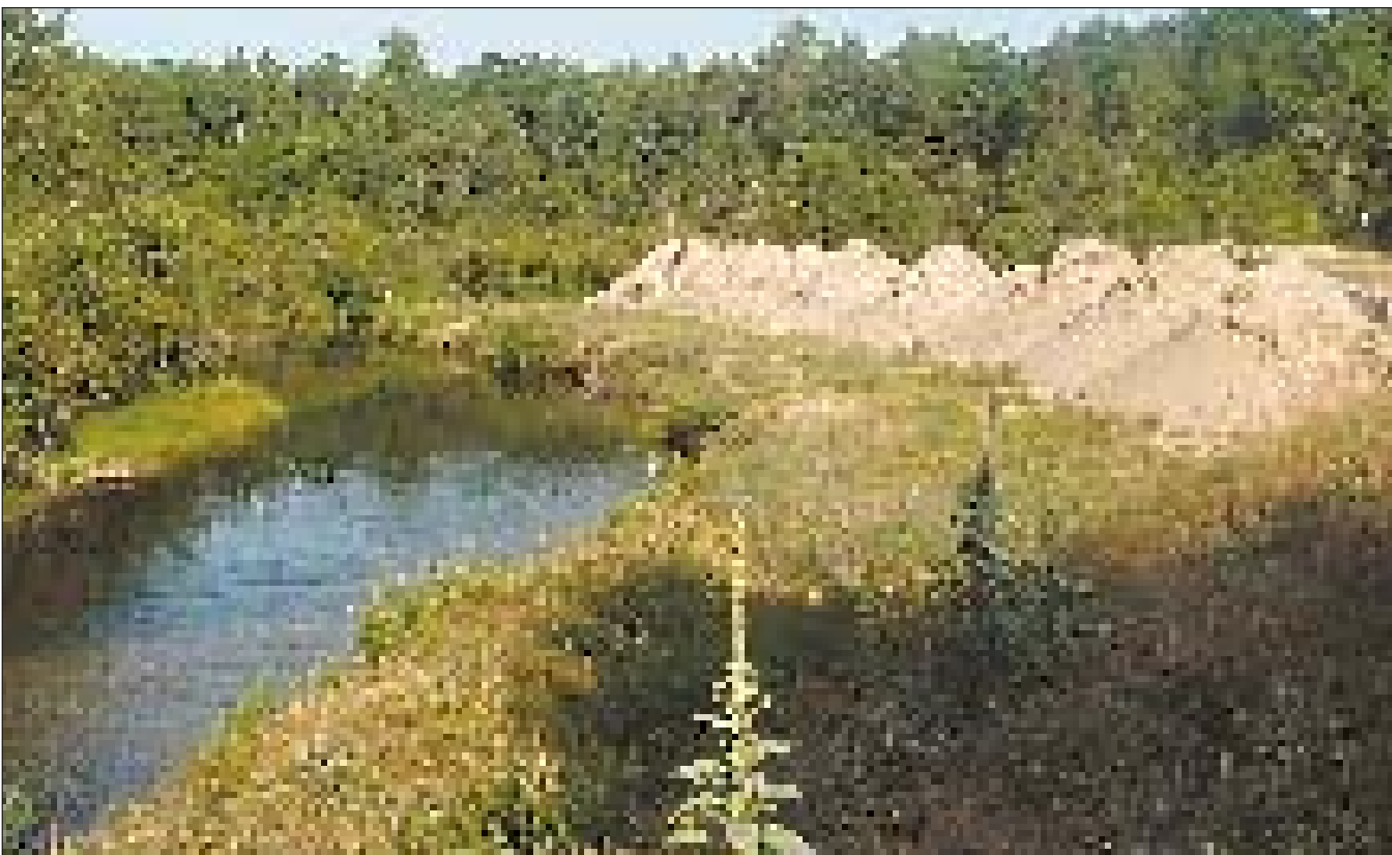
Mountains of sand — 90 dump truck loads — dredged from the north branch of the Boardman River “de-waters” before being moved. Since 1994, the Guernsey Lake sand trap alone has captured an estimated 6,000 cubic yards of sand from the river.
